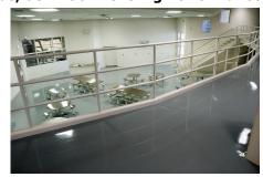
100% Solids, Semi-Self Leveling Performance Epoxy Floor
